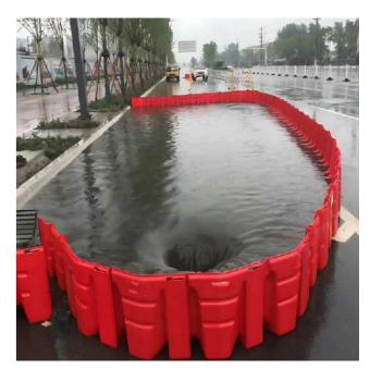
It works using the gravity of the water, pushing and holding the system on the ground.
